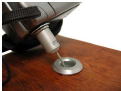
9. Tighten gently with security wrench.
